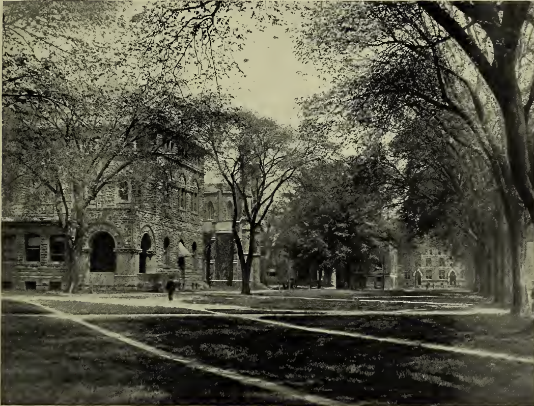
REAR VIEW OF CAMPUS, LOOKING SOUTH
